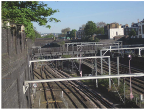
The 15 metre deep cutting will become 35m deep
