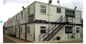
Seven works compounds near Camden Cutting
