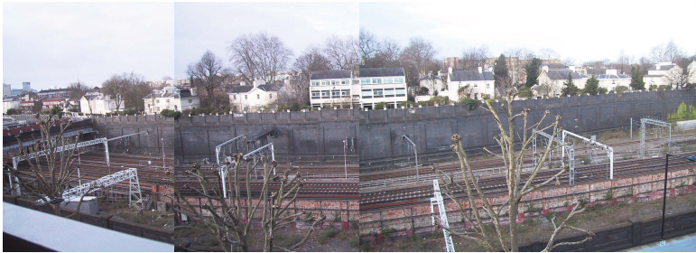
The 15 metre high retaining wall that will be demolished and rebuilt as 35 metres deep
