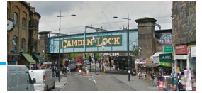
Nine North London Line bridges to be demolished & rebuilt
